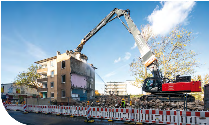
Scheidtweiler Str. 44-48 – Abriss November 2022
